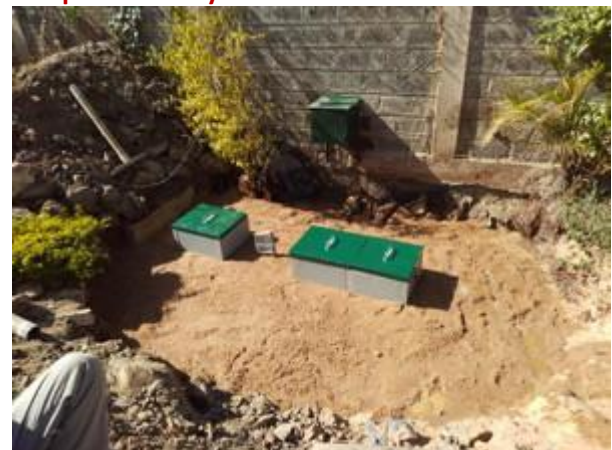
Step 4 – Completion, pending final landscaping
