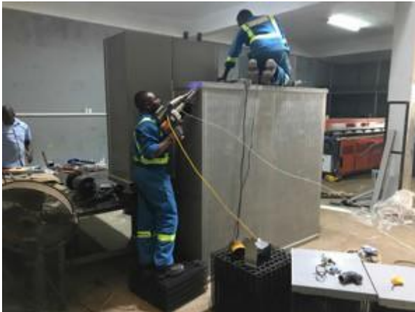
Step 1 – Tank Fabrication
